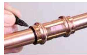
7B. Alternatively insert tube to tube stop and mark
