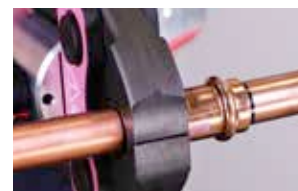
10. Complete the joint with the approved tool. Press once only
