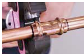
9. Align jaws squarely on the fitting
