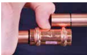
7B. Check the depth mark
