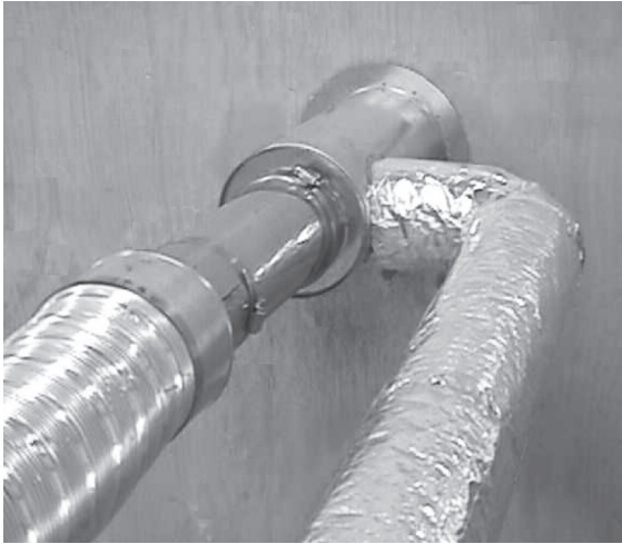
Figure 4 - Inside View of Vent Terminal
